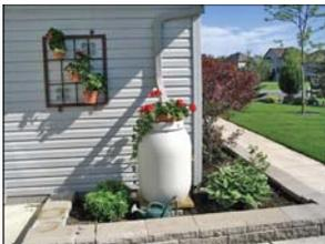
**Rain barrels are attached to downspouts which collect storm water running off your roof. An overflow system allows excess water to be directed elsewhere.**
